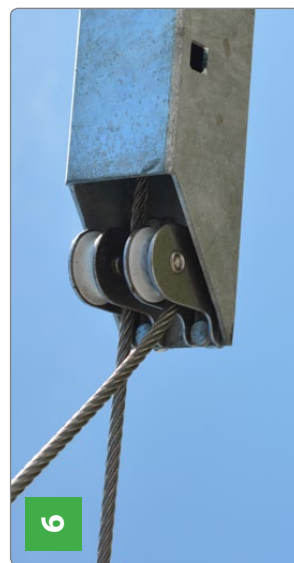
Wire rope to gate fitting. Plate and shackle fitted to module gate
