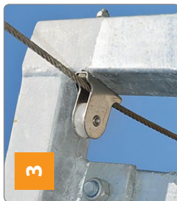
Draft module entrance. Pulleys bolted to module entrance frame
